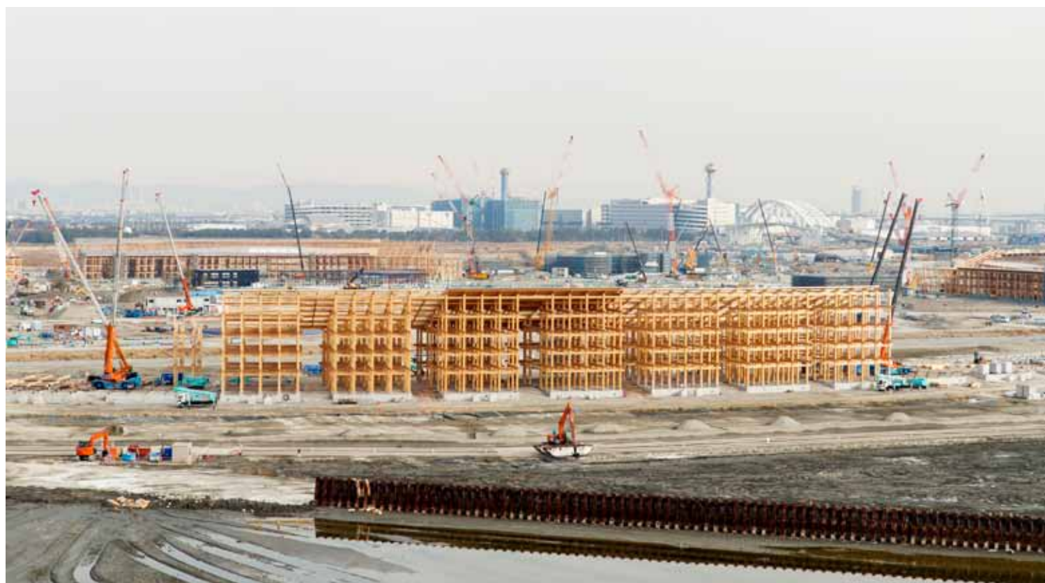
Venue under construction (EXPO 2025 Osaka/Kansai Expo)
