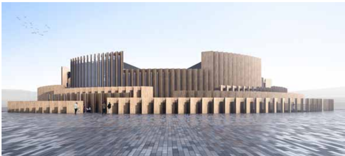
Completed image of the Japan Pavilion: Building using domestic CLT
